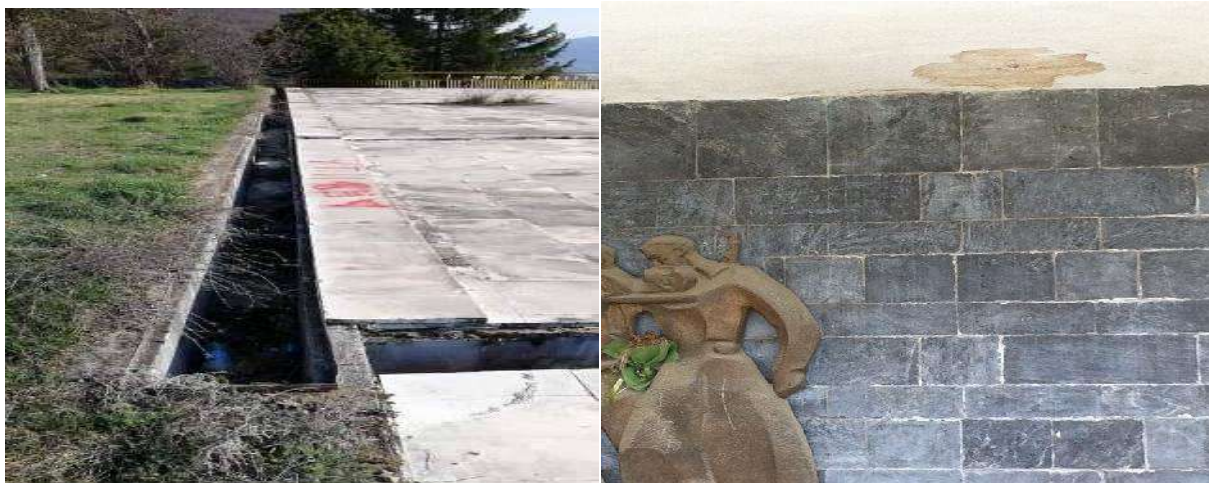
Figure13 Drainage channel for atmospheric watersFigure 14Damaged ceiling
