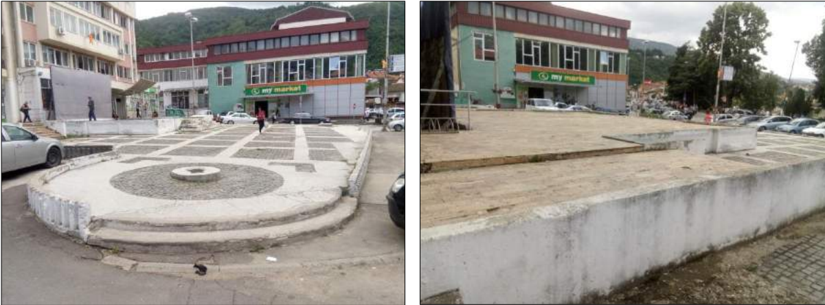
Fig. 3 - Current state of the stage on the square (obsolete, damaged and completely dysfunctional)
