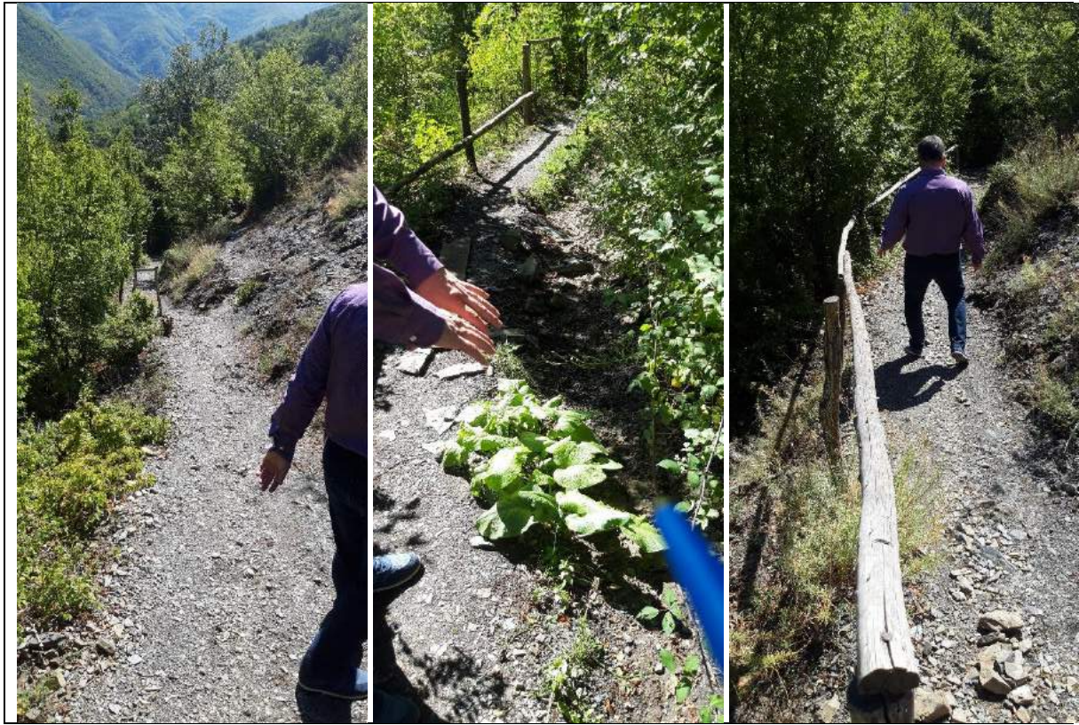
Figure 7: Appearance of an existing fence
