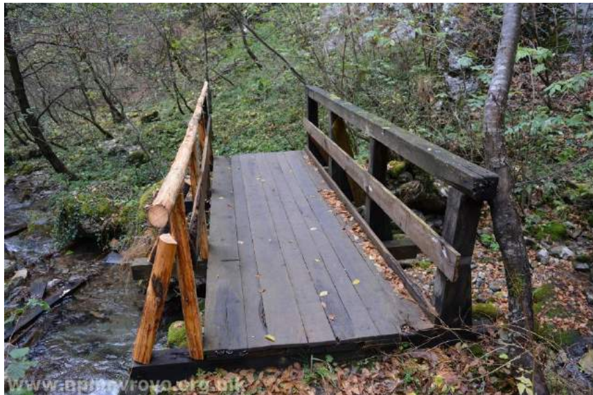
Picture 9: current situation on one of the bridges
