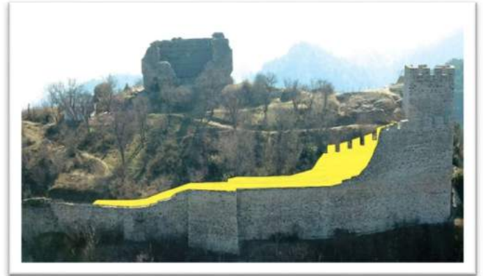
Picture 12: Outlook of the western rampart with the planned restoration marked in yellow
