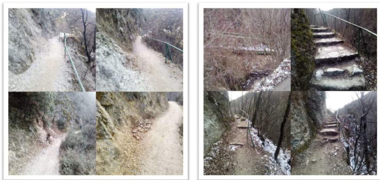
Picture 24: The current situation of the trim trail with the locations that will be landscaped
