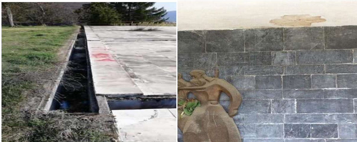
Figure13 Drainage channel for atmospheric watersFigure 14Damaged ceiling
