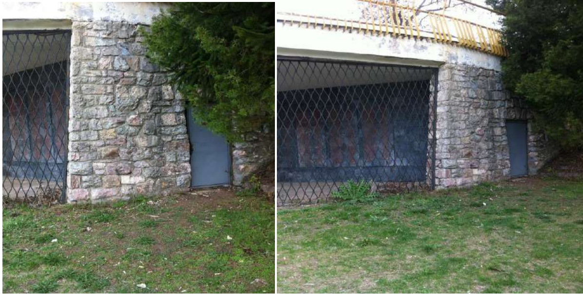
Figure11/12Door from the room where the relics are kept
