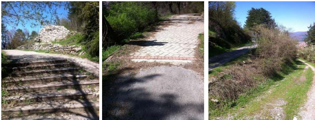
Figure 3 Remains of the medieval tower
