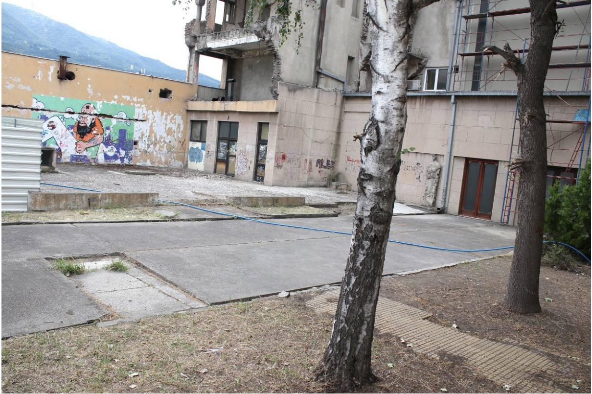
Existing condition: Photo 3
