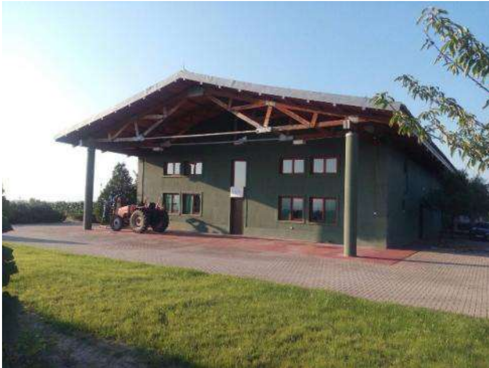
Figure 3. Lepovo – Current look. Adaptation works are applicable for the roof and the interior of the building.
