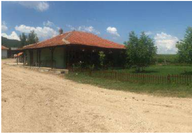
Figure 4. The tasting room in Barovo – Current look. Changes will be made to reconstruct Barovo site with wine barrel camp, a wine barrel kitchen, water supply station, etc.
