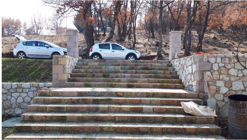
Figure 6 Location for installation of entrance door
